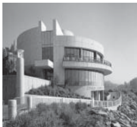
Foto 1 - Boathouse em Sawyer Point, Cincinnati, Ohio (PCI, 1989).
